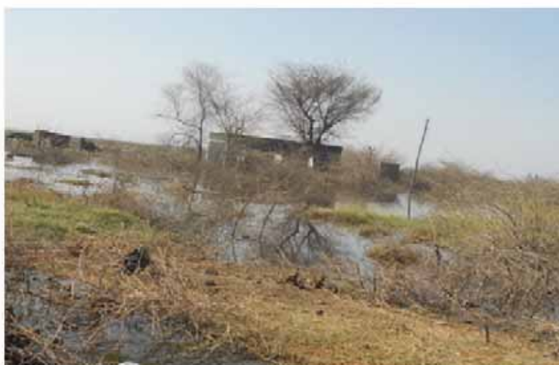
Figure 3. Fantalle floods destroyed the first high school built in the area.
